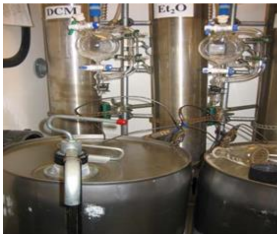
Figure 1: Bonding wires between drums
